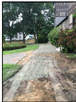
Front walkway underway
