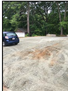
Parking lots ready for asphalt
